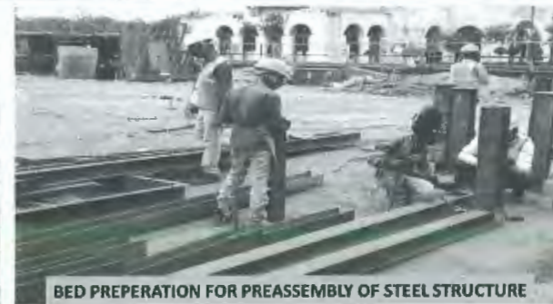
BED PREPERATION FOR PREASSEMBLY OF STEEL STRUCTURE
